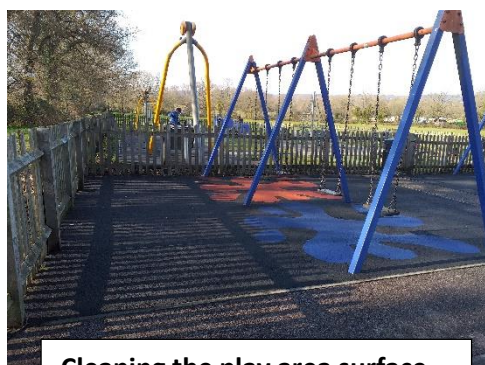
Cleaning the play area surface
