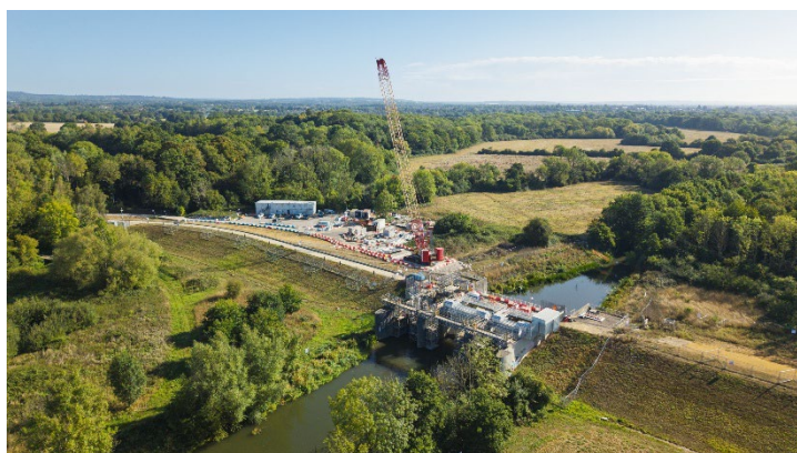
Above: Drone image of the Leigh construction site
