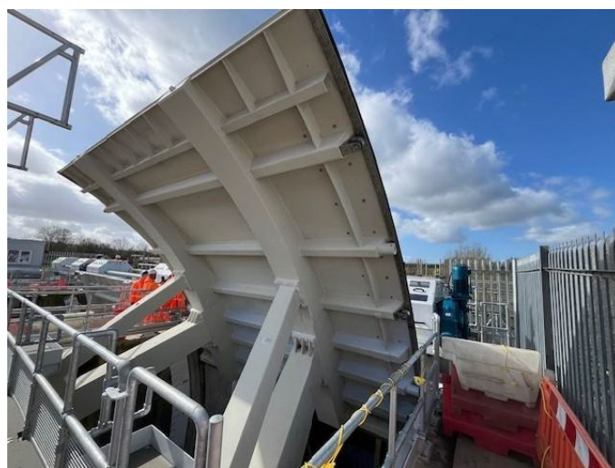
Above: North gate fully open during testing
