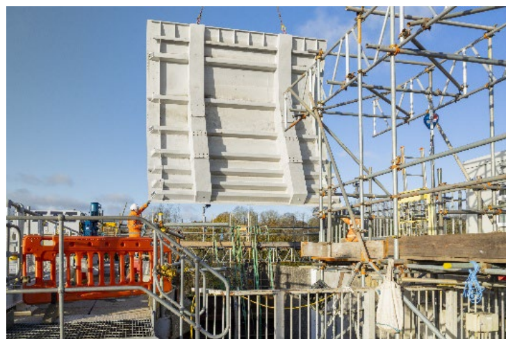
The north gate being lifted into the control structure
